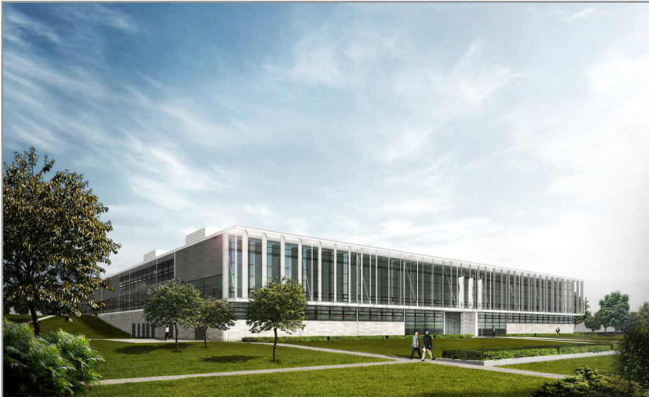
Investment in the future: The WITTENSTEIN Innovation Factory at the company's headquarters in Igersheim
